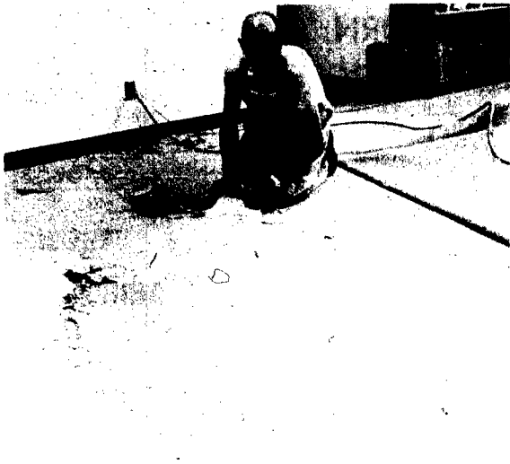
TEN YEAR VETERAN of the Wayne High maintenance staff, Al Ahlman, rips up the foam rubber backing of old carpeting in the library to make room for the new floor covering.
