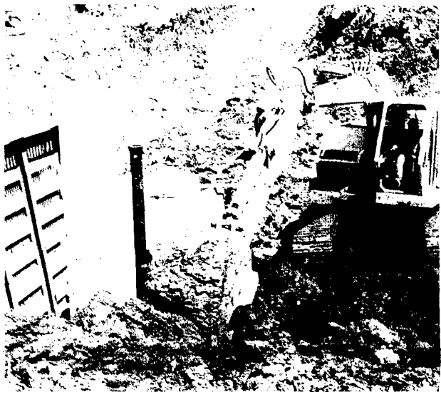
AN EMPLOYEE of the Midwest Bridge and Construction company, Norfolk, backfills a left station which is a part of the new sanitary sewer system being constructed this summer. The system is one of several projects underway in Wayne this summer.
